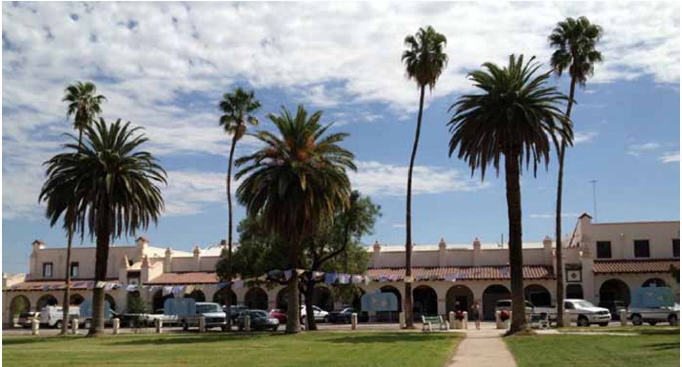
Arizona Economic Development Project
